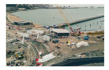
Tony Gee worked on the £115m Dover Western Docks revival Scheme for VolkerStevin Boskalis Westminster JV to design a new 500m long public access pier and navigation access structure and decking of quay walls.
